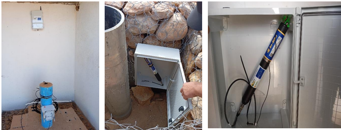
Figure 19. Installed sensors for water level and quality
